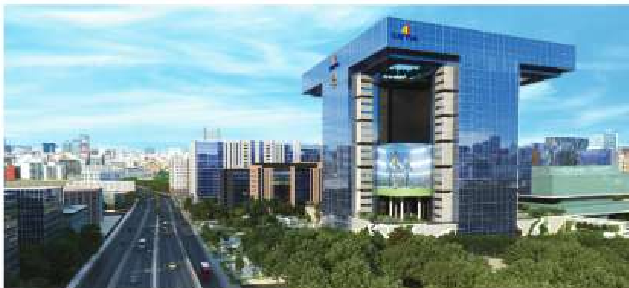
Inga Tower being developed on PPP model in association with the Telangana government.
