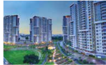
Greenage Hosur Main Road, Bengaluru
