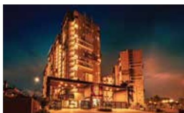
East Crest Near Budigere Cross, Bengaluru
