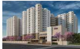
ASHRAYA Bengaluru-Mysuru Expressway Bidadi
