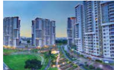
Greenage Hosur Main Road, Bengaluru
