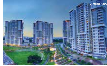
GREENAGE Hosur Main Road, Bengaluru
